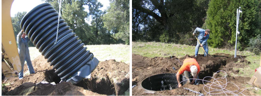
Figure 2-3. Construction of TA.BNLO using first generation vault.
